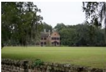
Front View of Middleton Place House
