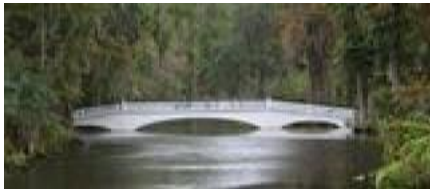
The White Footbridge
